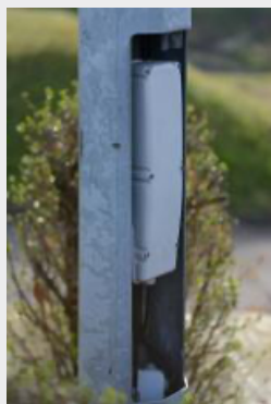
Inside of tower
