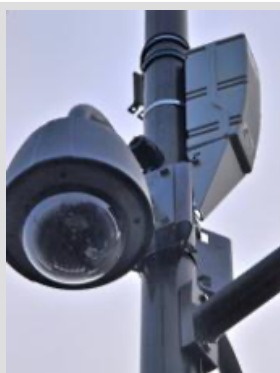
Top of tower
